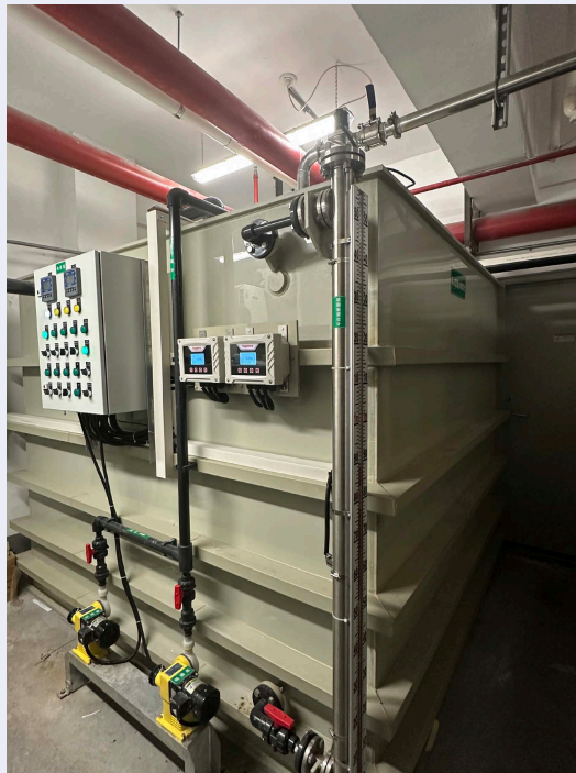
High-concentration wastewater catchment basin
