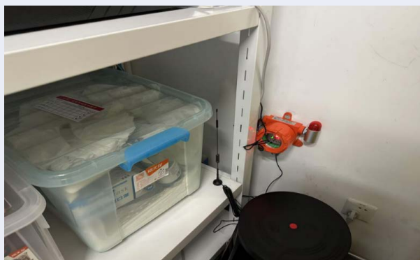
Pictured: Flammable gas alarm
